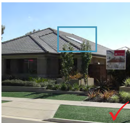
Figure 50 – Solar panels follow the roof pitch
