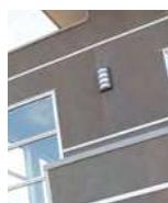
Lightweight Cladding types - flat panel
