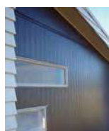
Lightweight Cladding types - vertical panel
