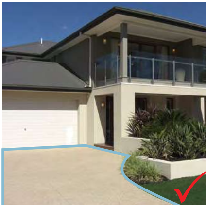
Figure 33 – Textured concrete surface
