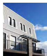
Lightweight Cladding types - corrugated and batted
