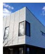
Lightweight Cladding types - corrugated and batted
