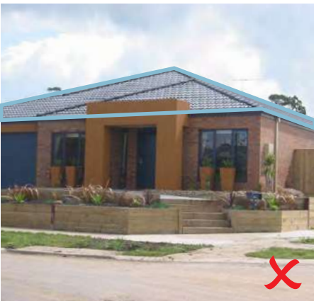
Figure 13 – Non compliant treatment to eaves
