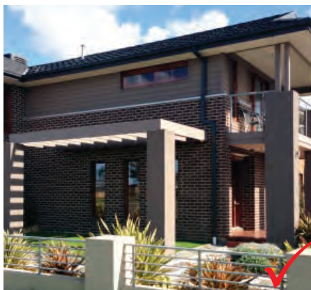
Figure 46 – Upper floor has sun protected from the eave and the lower floor from the pergola
