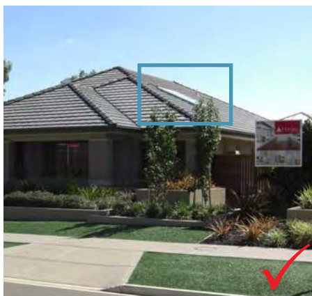
Figure 50 – Solar panels follow the roof pitch
