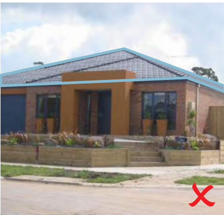
Figure 13 – Non compliant treatment to eaves
