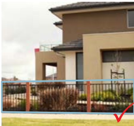
Figure 35 – Largely transparent front fencing
