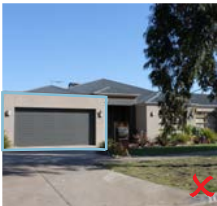
Figure 23 – Garage should be set back from the front wall
