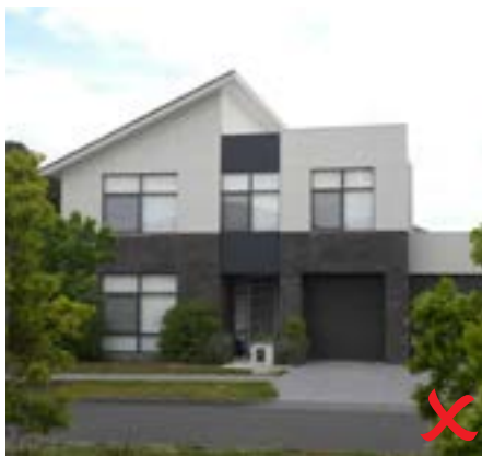
Figure 47 – North facing windows have no passive sun control
