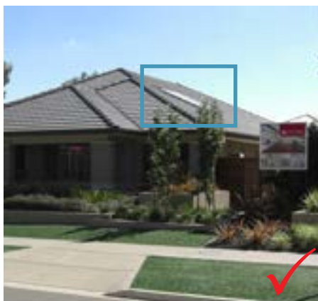
Figure 50 – Solar panels follow the roof pitch
