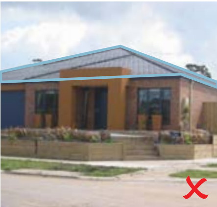
Figure 13 – Non compliant treatment to eaves
