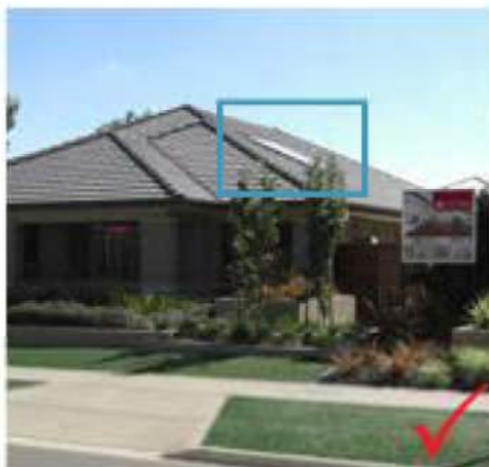
Figure 50 – Solar panels follow the roof pitch
