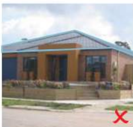
Figure 13 – Non compliant treatment to eaves
