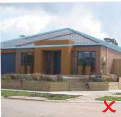
Figure 13 – Non compliant treatment to eaves
