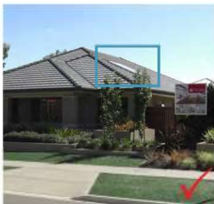
Figure 50 – Solar panels follow the roof pitch
