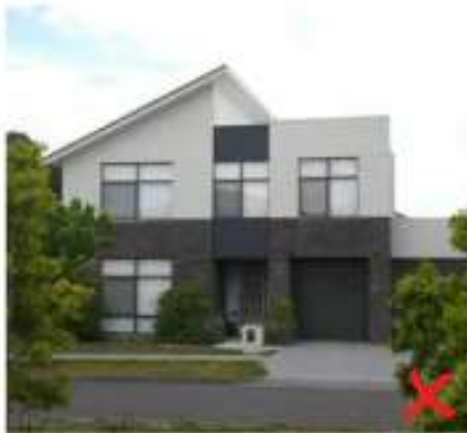
Figure 47 – North facing windows have no passive sun control
