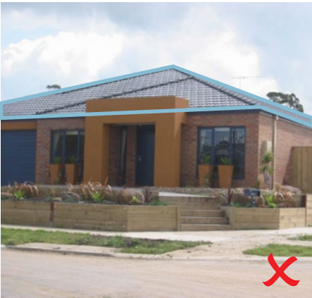
Figure 13 – Non compliant treatment to eaves
