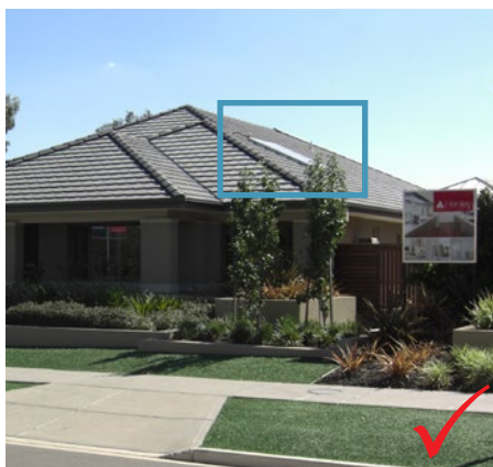
Figure 50 – Solar panels follow the roof pitch
