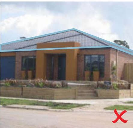
Figure 13 – Non compliant treatment to eaves
