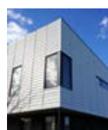
Lightweight Cladding types - corrugated and batted
