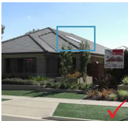
Figure 50 – Solar panels follow the roof pitch
