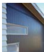
Lightweight Cladding types - vertical panel
