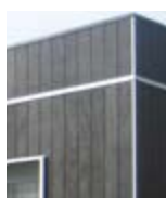
Lightweight Cladding types - vertical panel
