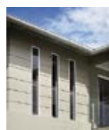
Lightweight Cladding types - horizontal panel
