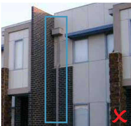
Figure 54 – Downpipes must not be on the front façade
