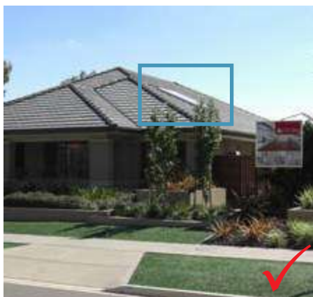
Figure 50 – Solar panels follow the roof pitch
