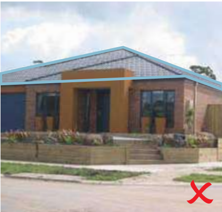
Figure 13 – Non compliant treatment to eaves
